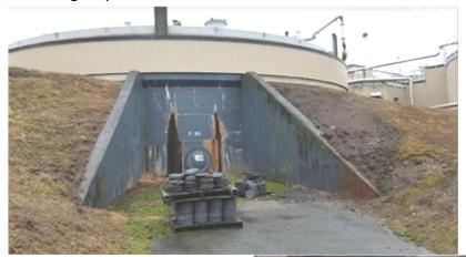
Photo on left: Access door of the Secondary Digester, showing obvious signs of needed repair.
