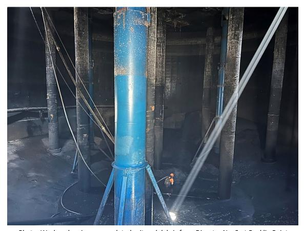
Photo: Worker cleaning accumulated grit and debris from Digester No. 3 at Bucklin Point.
