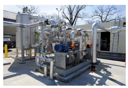
Photo: Packaged chiller Heat Exchanger and Primary Digester Blowers.
