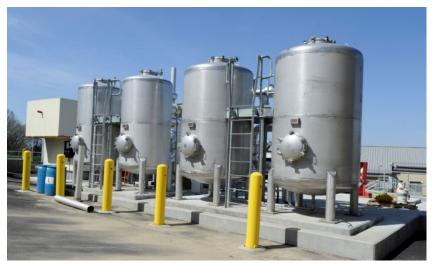
Photo: Biogas Conditioning Filter System. The biogas needs to be treated before it is fed to the engine. Excess moisture is removed from the biogas. Two filters remove siloxanes, and two filters remove hydrogen sulfide.
