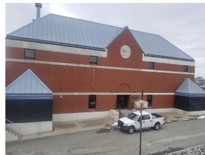
FPWWTF Ernest Street Pump Station
