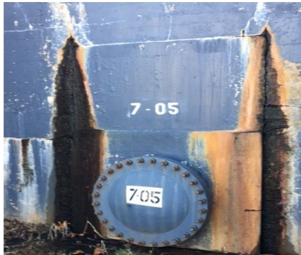
Photo: Secondary Digester
