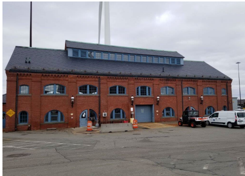
Photo: Existing FPWWTF Maintenance Building
