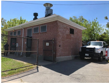
Reservoir Avenue Pump Station
