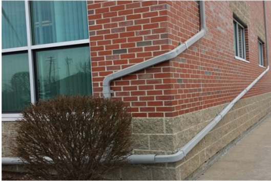
Photo: Downspouts at NBC's Corporate Office Building
