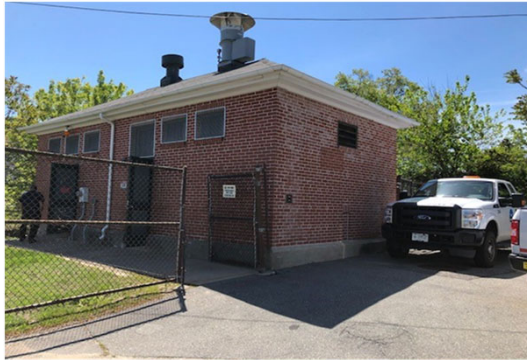
Photo: Reservoir Avenue Pump Station
