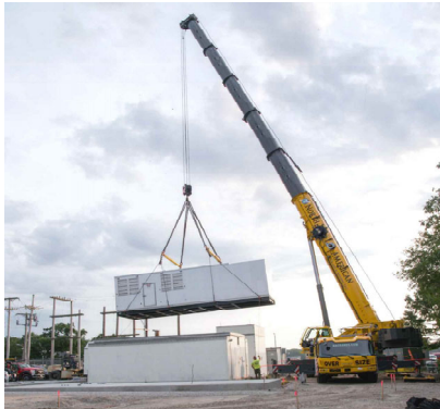
Photo: 2,000 kWh Generator Installation
