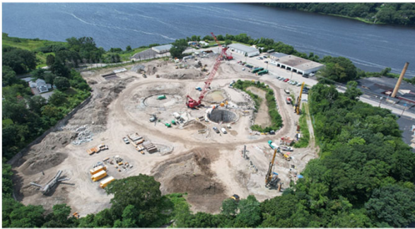
Photo: Pawtucket Tunnel Site
