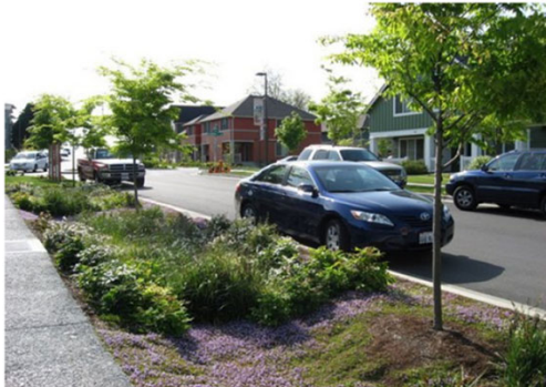
Photo: Example of Green Stormwater Infrastructure
