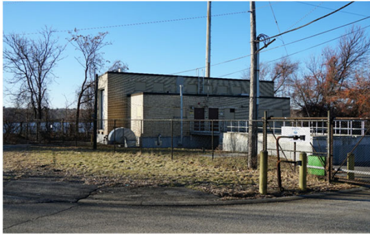
Photo: Omega Pump Station
