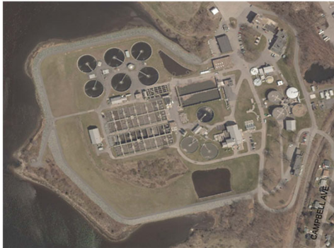
Photo: Existing Clarifiers at Bucklin Point
