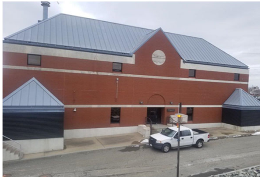
Photo: Ernest Street Pump Station
