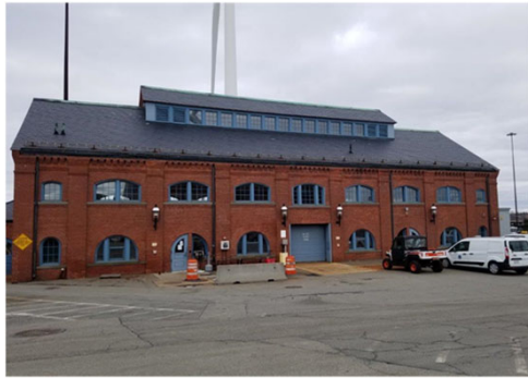
Photo: Existing FPWWTF Maintenance Building
