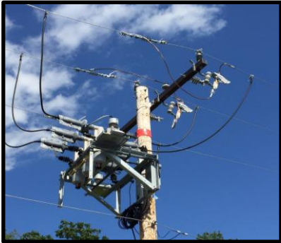
Protective & Sectionalizing: Vacuum Circuit Recloser
