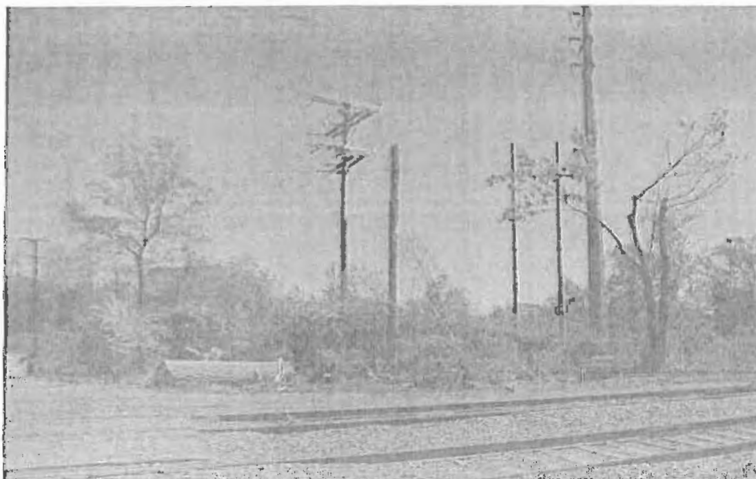
04. SE Quadrant and Overhead Lines
