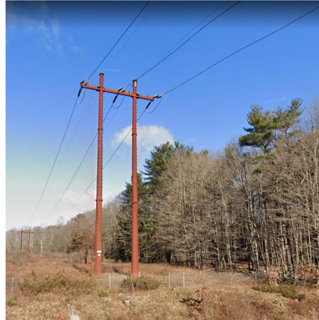
Proposed Structure Steel H-Frame
