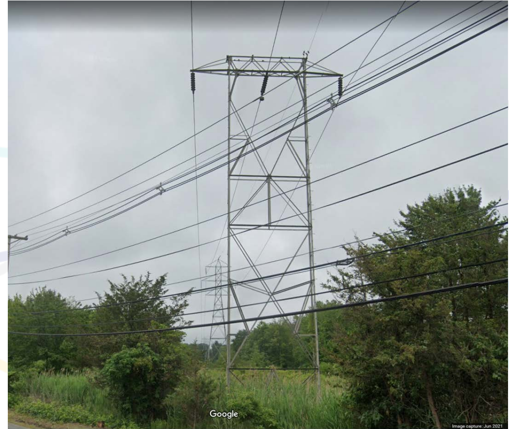
View South – George Washington Highway, Lincoln
