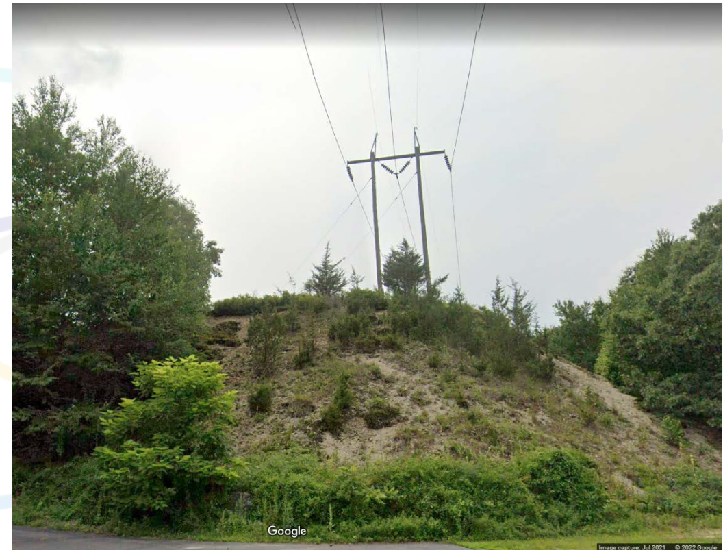
View to West – River Road, Lincoln
