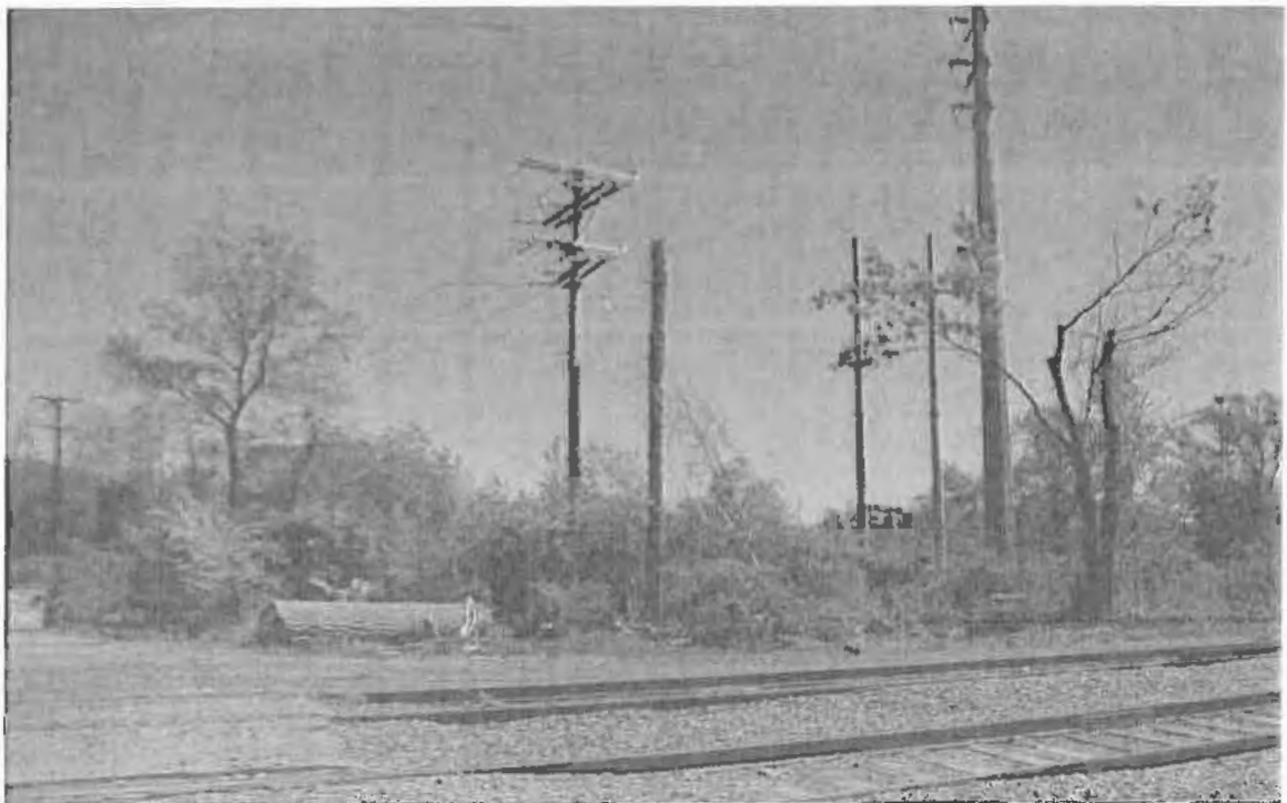
04. SE Quadrant and Overhead Lines
