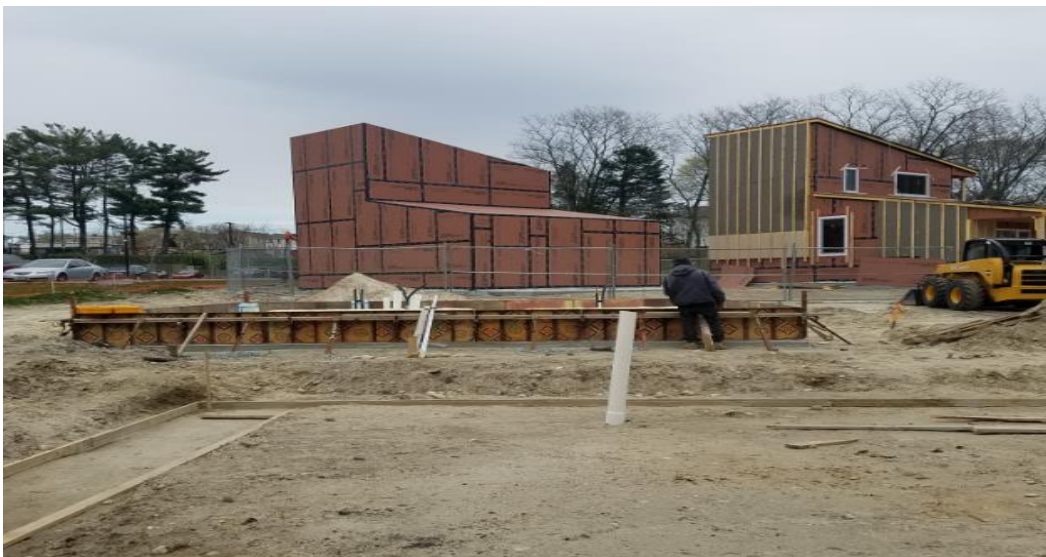
Pictured above: Sheridan Small Homes, Under Construction
