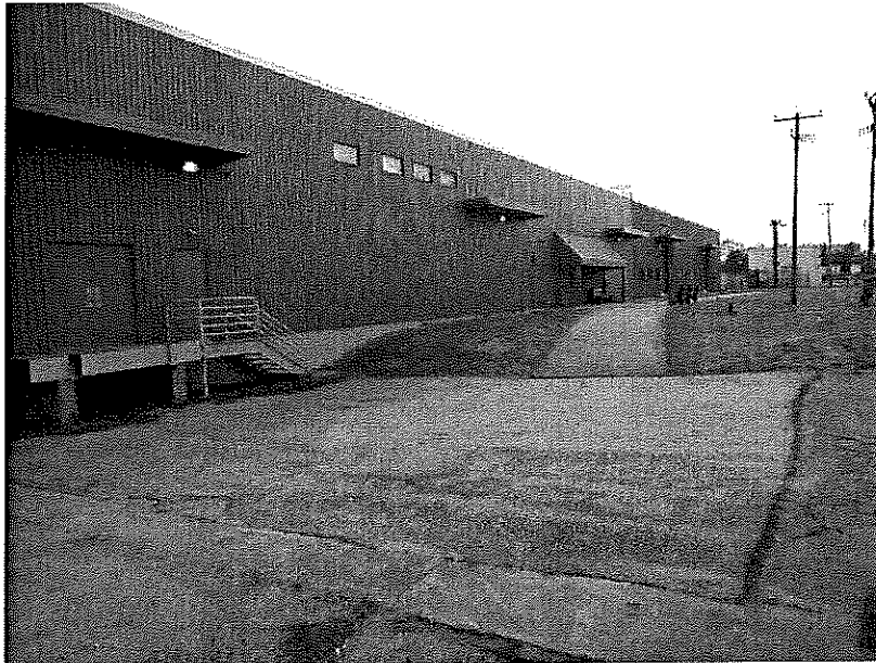
Photo A-4: Typical metal building façade (north wall)
