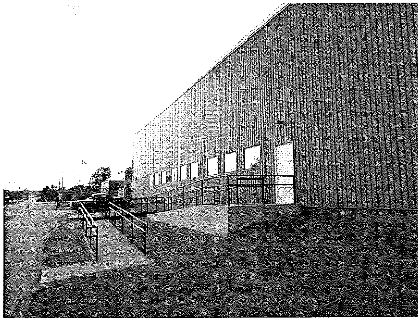
Photo D-8: Main building – South wall (looking west)
