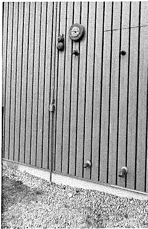
Photo B-51: Water Motor Alarms, Drains and Post-indicator valve (Typical)
