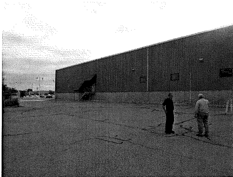
Photo D-6: Main building – East wall
