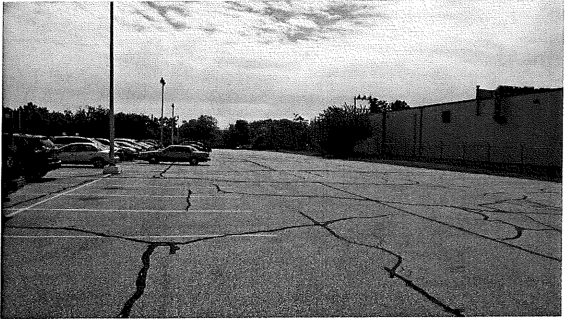
D-13: Southern parking lot surface
