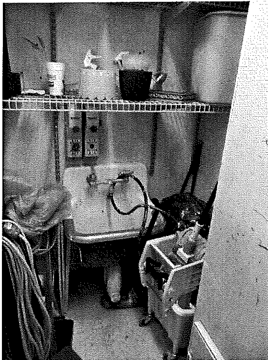
Photo B-10: Janitor Closet Mop sink
