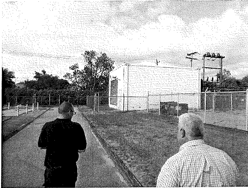
Photo A-9: Generator House
