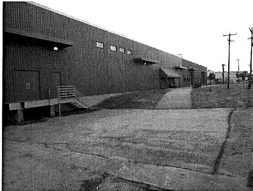
Photo D-4: Main building – North wall
