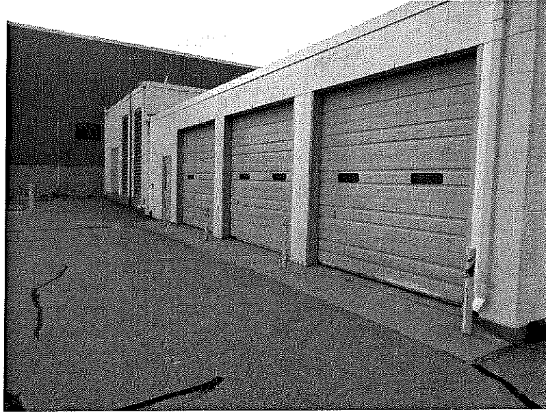
Photo A-7: Concrete masonry façade at garage in north eastern corner
