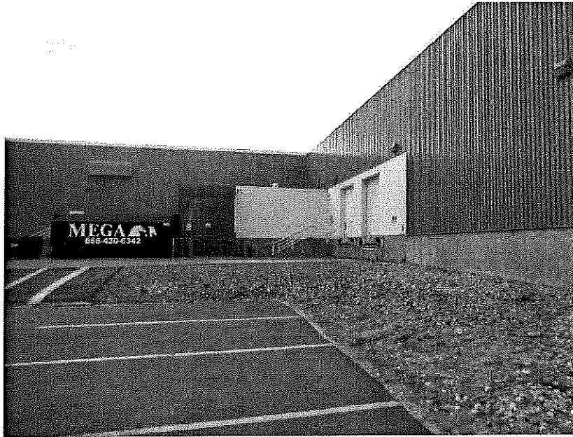
Photo A-8: Concrete masonry façade at southeastern loading dock
