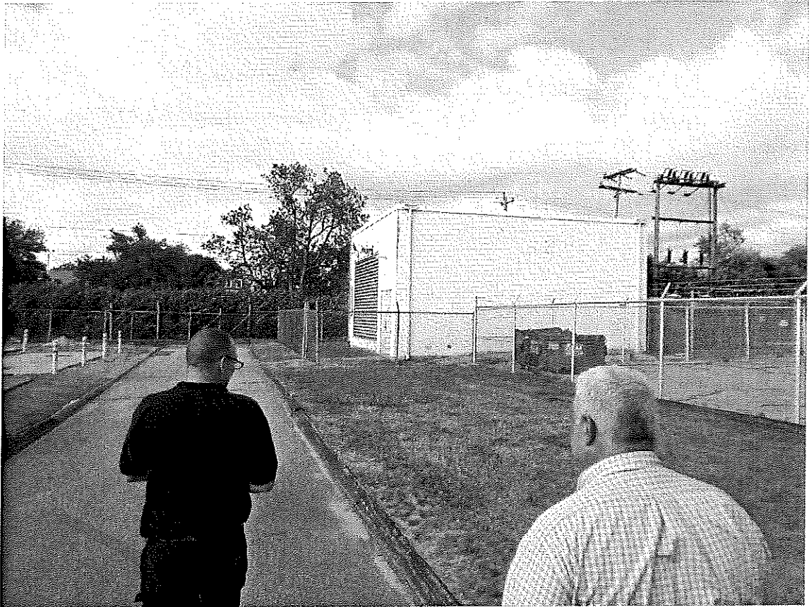
D-9: Generator house – South face (looking north)
