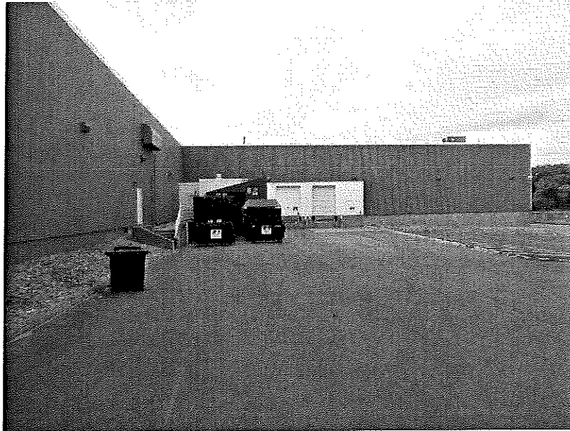
Photo D-7: Main building – East side (looking north)
