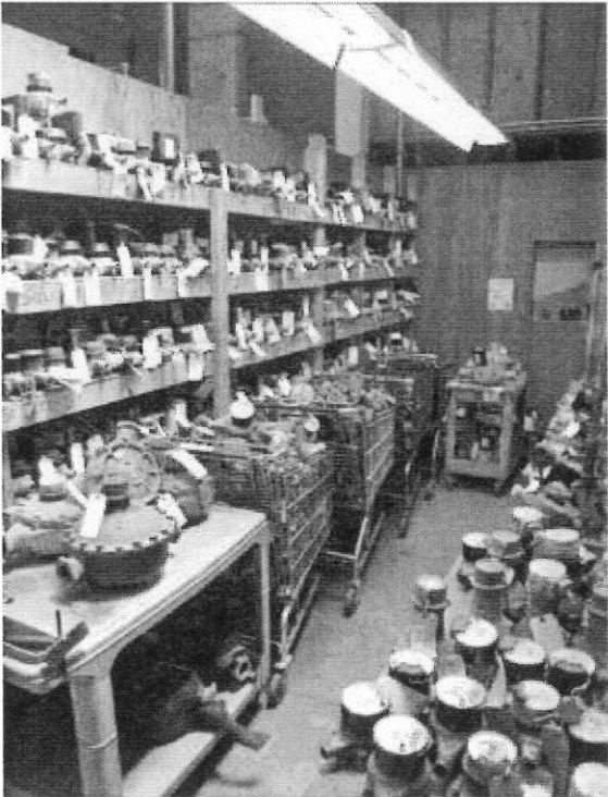
Providence Meter Room
