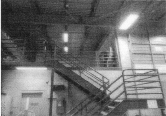
VIEW OF STORAGE MEZZANINE SPACE OVER FRONT GARAGE FOR FORMER ARMORED TRUCKS
