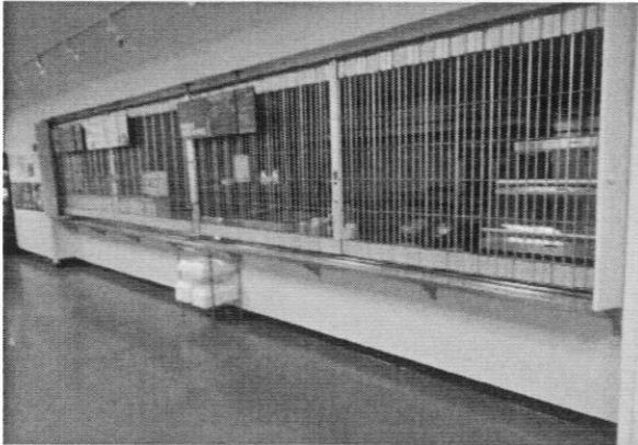
VIEW OF FORMER VAULT ROOM
