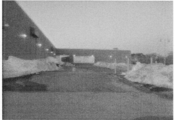
EASTERLY SIDE VIEW; GARAGE AT REAR LOOKING NORTH
