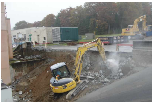
Excavation of slope for new wash water pipe
