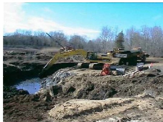
Sludge lagoon dredging operations in progress
