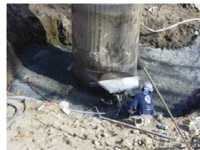
Removal of old East Portal Structure
