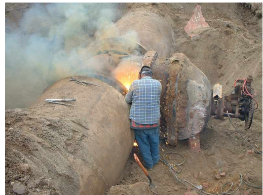
Removal of old 48 inch transmission gate valve
