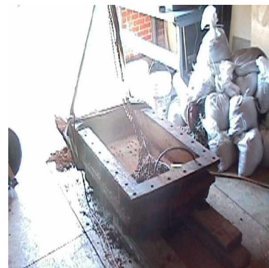
Old Longview Reservoir sluice gate being removed
