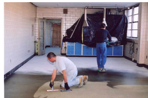
Installation of a new epoxy floor in the lab
