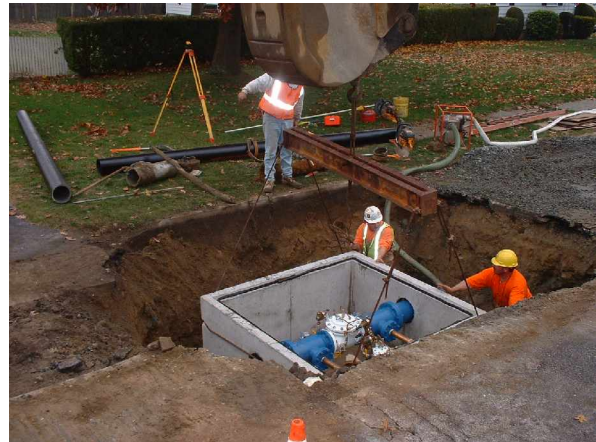
Installation of Pressure Reducing Valve Station
