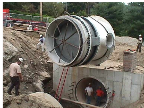
Lowering the 102" valve into place
