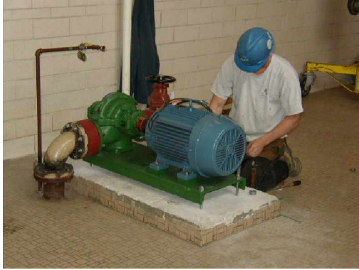
Wiring new service water pump
