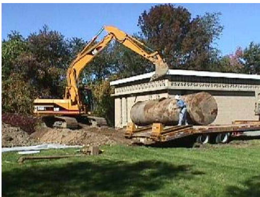
Removal of old underground fuel storage tank at the Aqueduct Pumping Station
