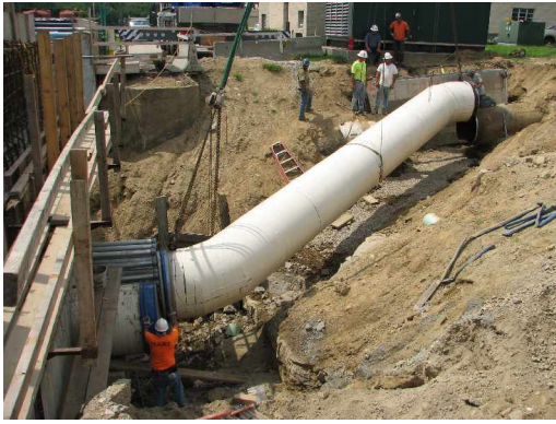
Installation of new 48 inch wash water pipe
