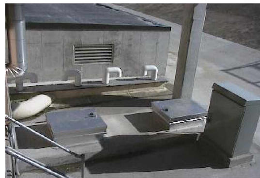
New access hatches and instrumentation panel installed over the opening of the venturi meters
