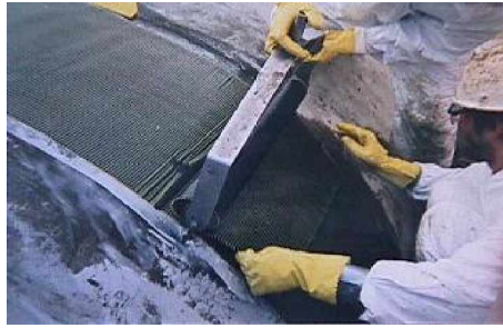
Application of carbon fiber to exterior of deteriorated section of 102" Aqueduct
