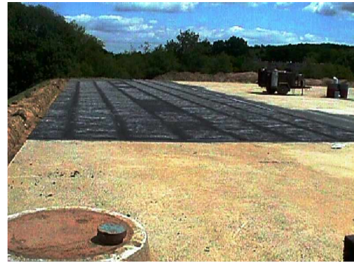
Aqueduct Reservoir Waterproofing
