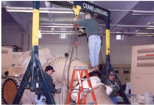
Installation of spool piece after valve installation
