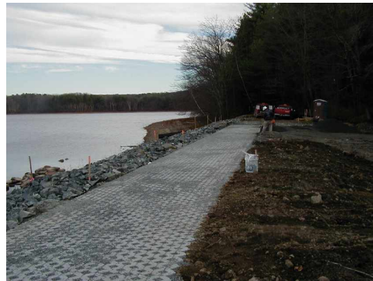
Regrading the access road on the crest of the dam
