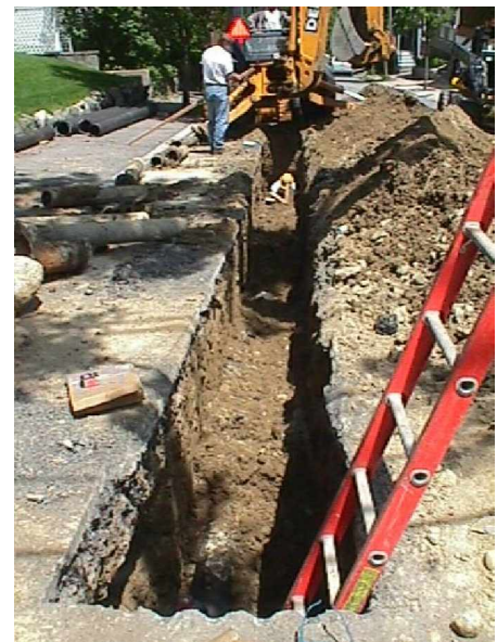
Main Replacement Work in Progress
