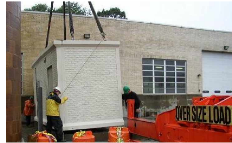
Lowering section of new blower building into place
