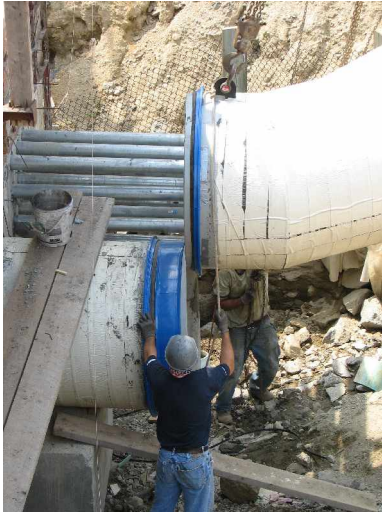
Installation of new 48" wash water pipe
