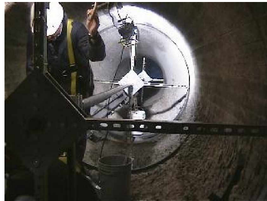
Concrete reconstruction and installation of new instrumentation in treatment plant's 72" x 42" effluent venturi meter
