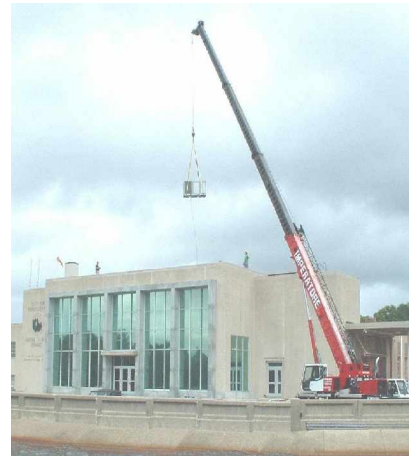
Placing A/C unit on top of the Auditorium
