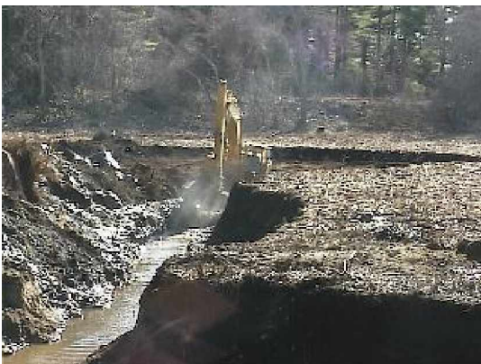
Sludge lagoon at the beginning of dredging operations
