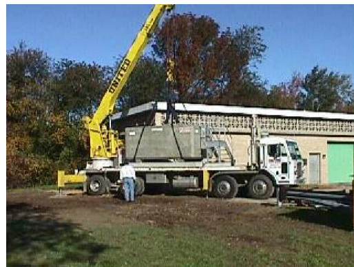
Delivery of new above ground fuel storage tank at the Aqueduct Pumping Station
