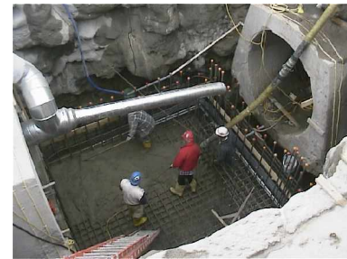
Pouring base slab of new valve enclosure
