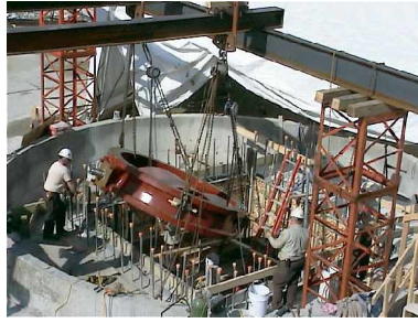
Lowering the 90” valve into place
