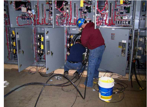
Installation of new motor control center
