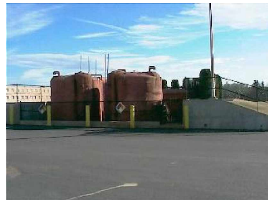
New liquid ferric sulfate bulk storage tanks
