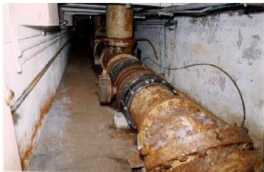
Neutaconkanut Pump Station piping before rehabilitation
