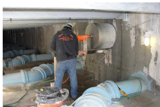
Coring for new wash water pipe
