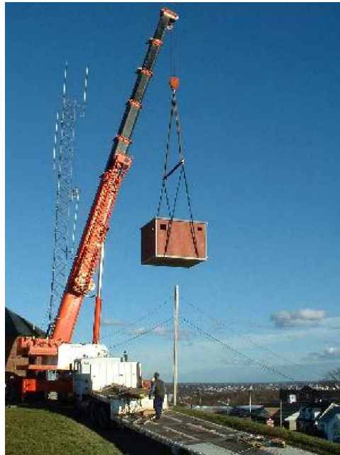
Lowering Communications Shed to Foundation
