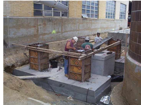
Footings for new access stairs to silos
