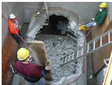
Opening into Aqueduct at New Access Structure
