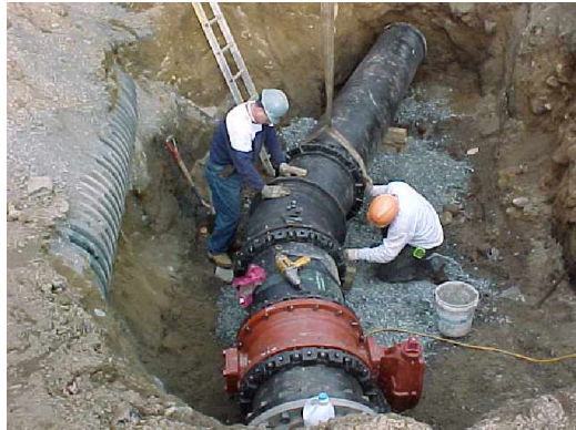
Installation of 24" main on Conley Avenue
