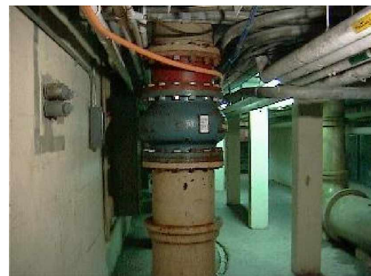
New check valve installation
