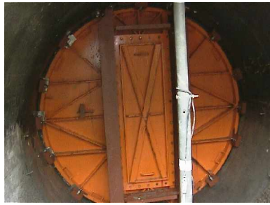
90” disc plug in place prior to rehabilitation and valve installation
