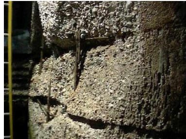
Extensive concrete corrosion damage in vicinity of south venturi meter
