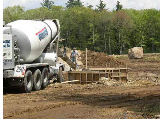
Concrete pour of wing wall on culvert sections for residual management system
