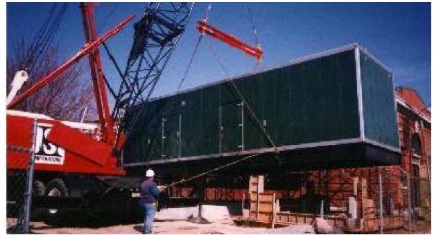
Delivery of new generator enclosure
