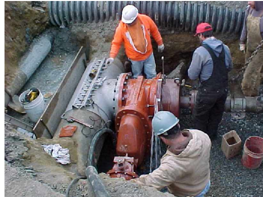
Installation of 24" tapping sleeve and valve
