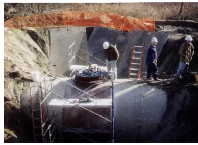
Installation of new access manhole into 102" Aqueduct
