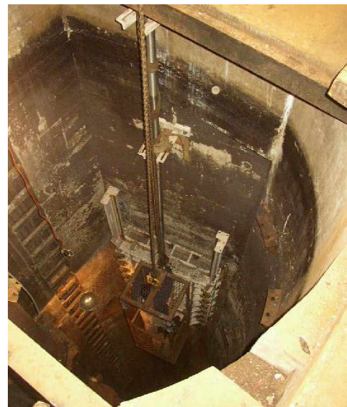
Installation of new sluice gate
