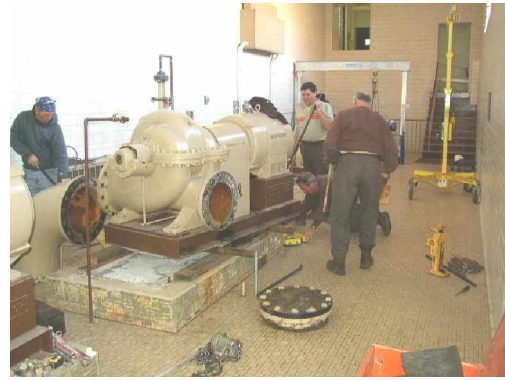
Removal of existing Wash Water pump
