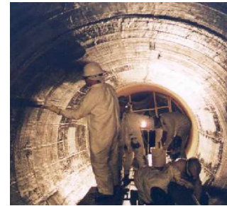
Crew applying carbon fiber lining to interior of deteriorated section of 102" Aqueduct
