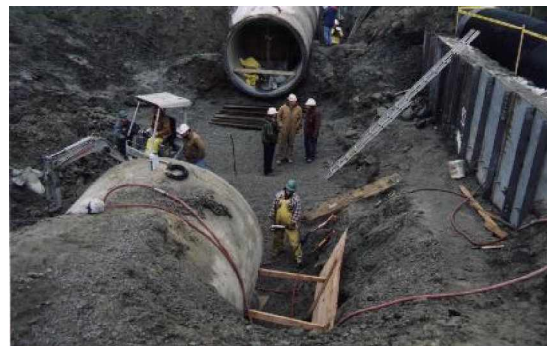
102" Aqueduct prepared for replacement sections
