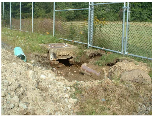
Section of vitrified clay pipe replaced with PVC
