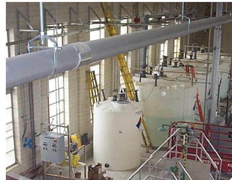
New fluoride tanks in place
