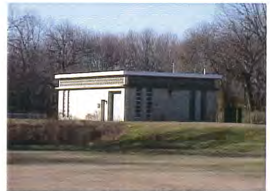
Aqueduct Reservoir Pump Station
