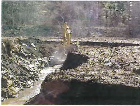
Sludge lagoon at the beginning of dredging operations
