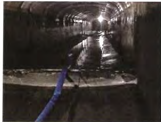
Interior of the Clearwell
