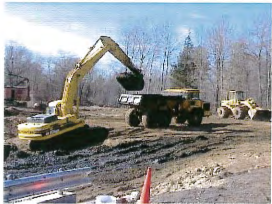
Sludge lagoon dredging operations in progress
