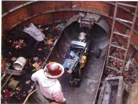
Interior cement mortar lining machine in 48" steel transmission main
