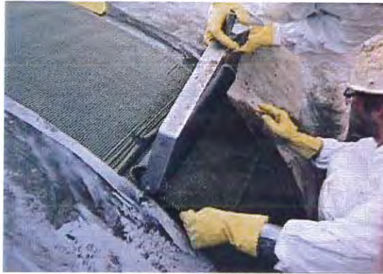
Application of carbon fiber to exterior of deteriorated section of 102" Aqueduct
