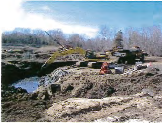
Sludge lagoon dredging operations in progress
