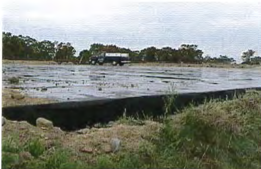
Rehabilitation and waterproofing of Longview Distribution Reservoir roof slab
