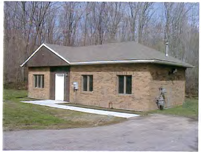
Dean Estates Pump Station
