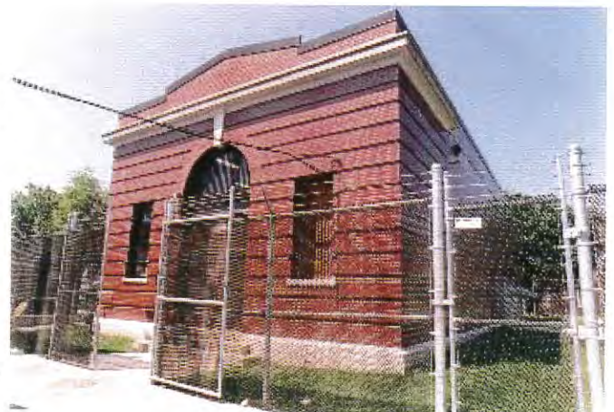
Bath Street Pump Station
