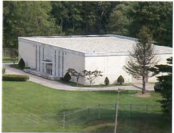
Raw Water Pumping Station
