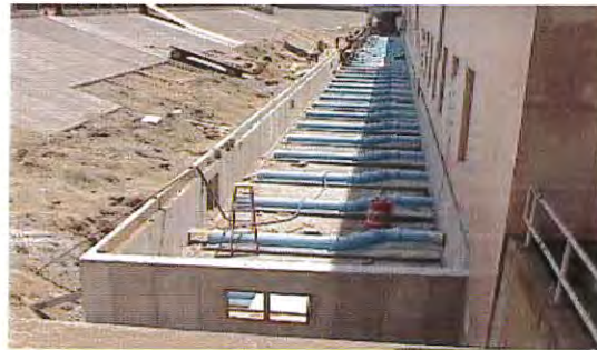
Construction of clearwell protective structure
