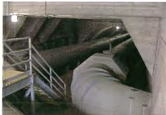
Twin 60 inch mains after rehabilitation
