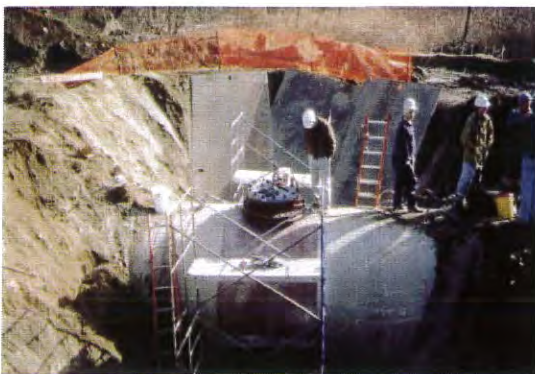
Installation of new access manhole into 102" Aqueduct
