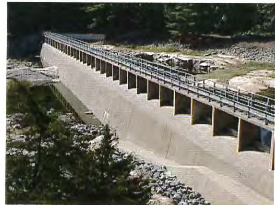
400 foot Gainer Dam spillway showing new concrete facing
