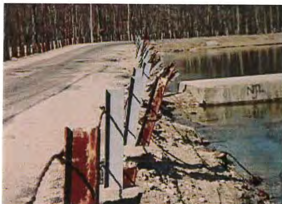
Ponaganset Reservoir before rehabilitation
