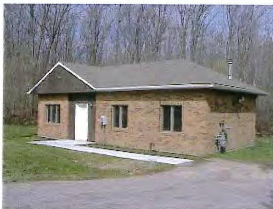
Dean Estates Pump Station
