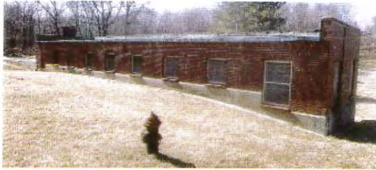
Exterior of Neutaconkanut Pump Station before rehabilitation
