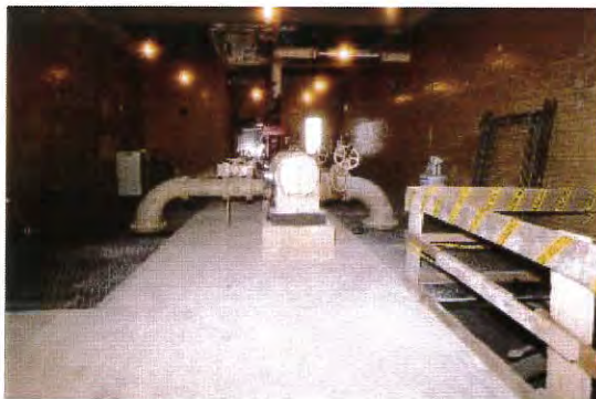
Bath Street Pump Station before upgrade
