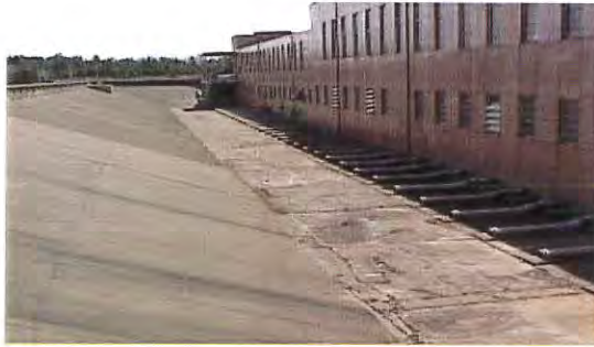
Effluent clearwell yard at treatment plant prior to rehabilitation
