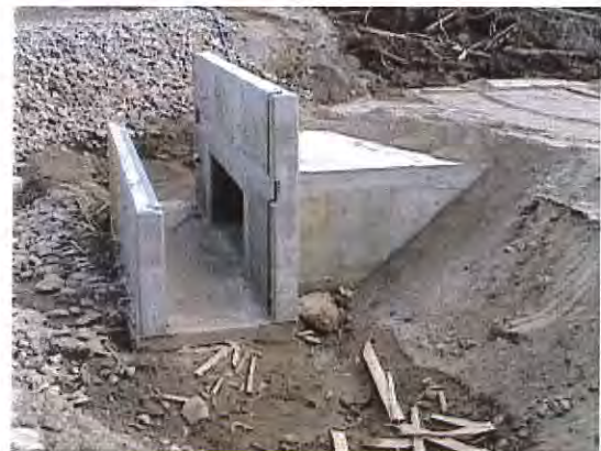
New culvert and stop-log structure prior to final backfill
