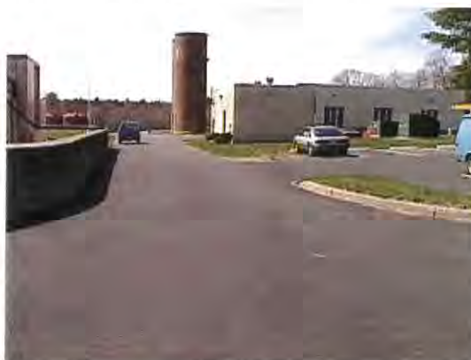
Rehabilitated north Access Road to treatment plant
