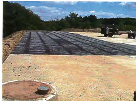
Rehabilitation and waterproofing application on top of Aqueduct Distribution Reservoir
