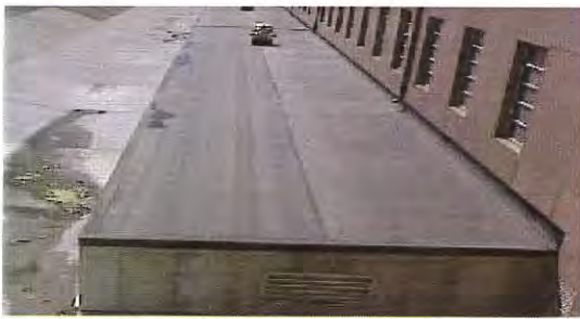
Completed clearwell protective structure
