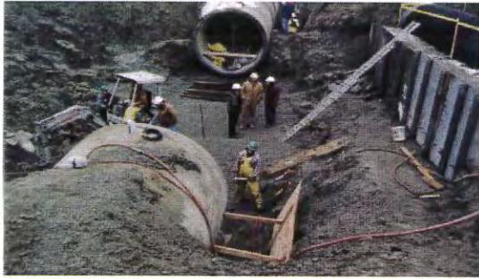
102" Aqueduct prepared for replacement sections
