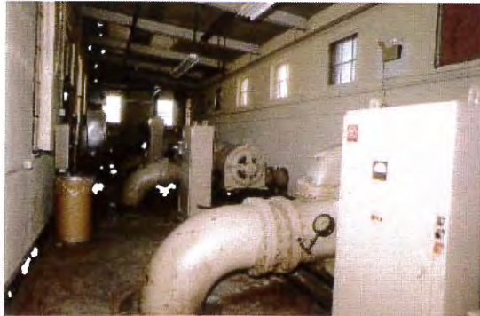
Interior of Neutaconkanut Pump Station before rehabilitation
