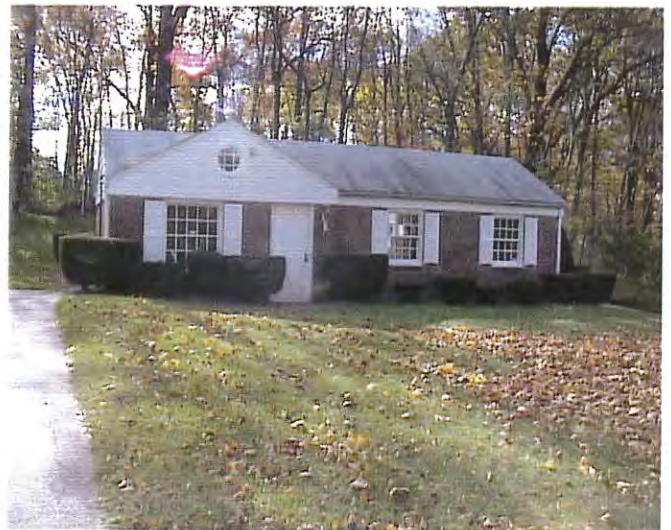
Garden Hills Pump Station
