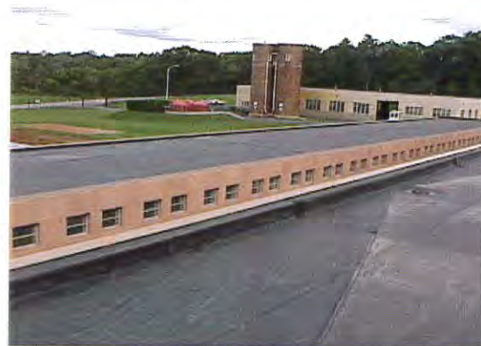
New treatment plant replacement roof
