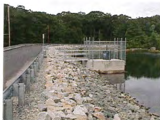
Ponaganset Reservoir after rehabilitation
