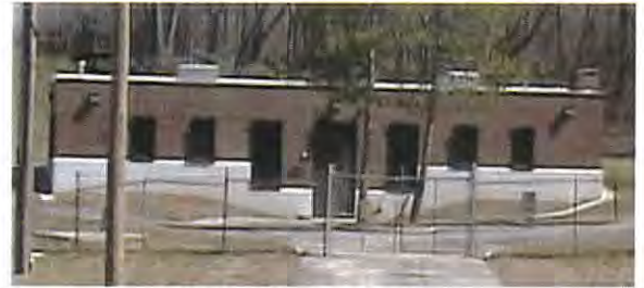
Neutaconkanut Pump Station
