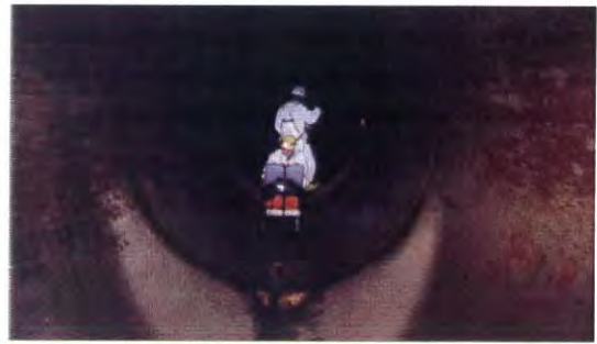
Impact Echo testing of 102" Aqueduct from interior
