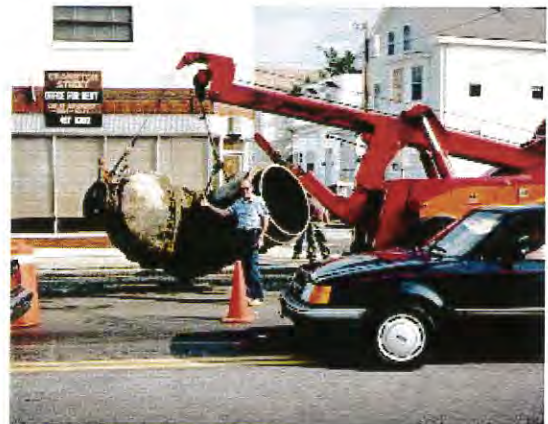
Removal of old 42 inch transmission gate valve
