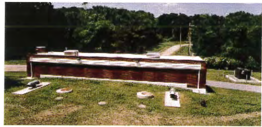
Exterior of Neutaconkanut Pump Station after rehabilitation
