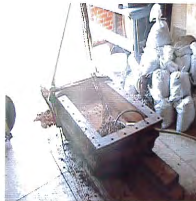
Old Longview Reservoir sluice gate being removed
