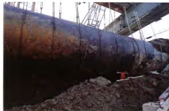
Temporary supports to adjacent 66" transmission main
