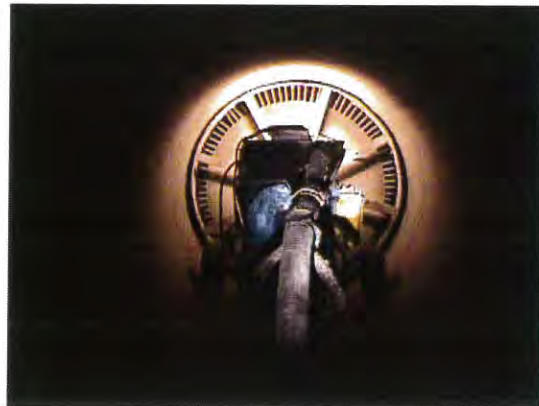
Lining machine applying and troweling cement mortar in 48" steel transmission main
