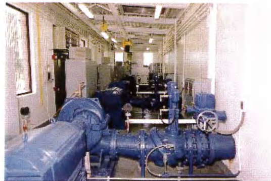
Interior of Neutaconkanut Pump Station after rehabilitation
