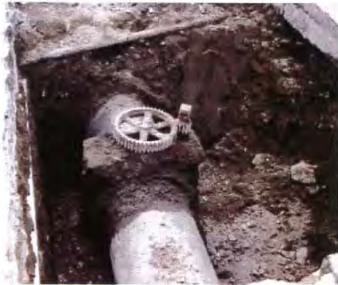
Antiquated 16 inch transmission gate valve prepared for replacement
