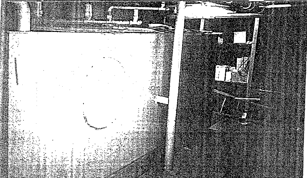
15/Void #5 w/ storage and bises water tank
