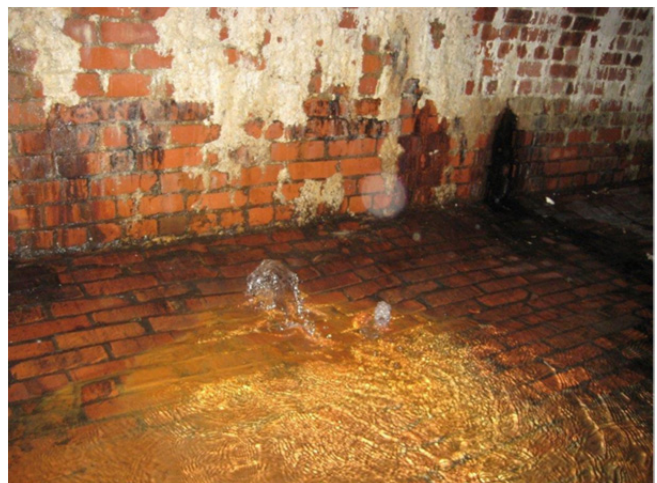
Phase II CSO Facilities WCSOI North Infiltration into existing WCSOI North overflow
