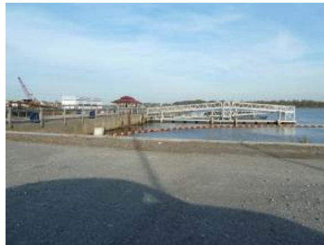
View of Pier (Photo Taken on November 7, 2011)
