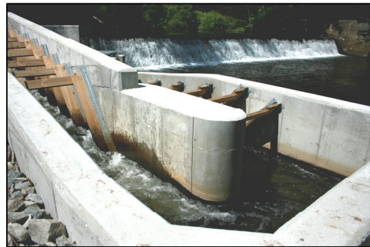
Fish ladder at Rising Sun Mills dam located in Providence.
