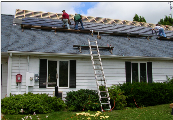
Photovoltaic shingles on the roof of the URI College of the Environment and Life Sciences Outreach Center.
