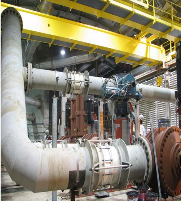
A view from the second floor slab of the Tunnel Pump Station. A 20 ton crane (yellow) has been incorporated within the cavern in order to access and properly maintain the various pumps, piping, and valves.
