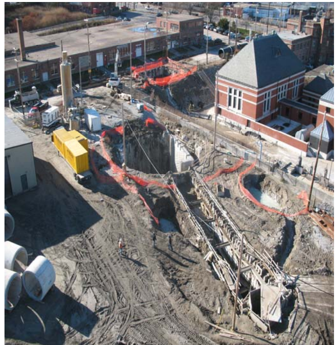
The 067 outfall which is 110" in diameter and the gate and screening structure which will carry the wet weather flow to the tunnel, then the Pump Station, to the Field's Point Wastewater Treatment Facility.
