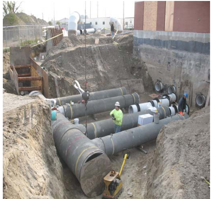
The Pump station Force Main, consisting of a header and 4 discharge pipes. The pipes carry the flow from the Tunnel Pump Station to the Field's Point Wastewater Treatment Facility.
