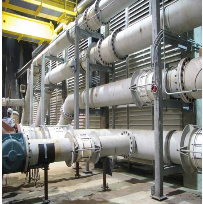
An interior view of the 4 separate discharge pipes which carry the flow from the Pump Station to the Force Main and finally to the FPWWTF.
