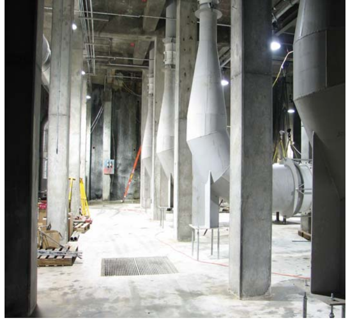
A view of the suction piping from the Pump Station's first floor slab, approximately 300 feet underground.
