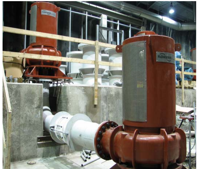
One pair of the 2 stage pumps, on the second floor slab of the Tunnel Pump Station. There are 4 sets of 2 stage pump pairs. Each pump is 400 HP and capable of pushing the flow up 300 feet.
