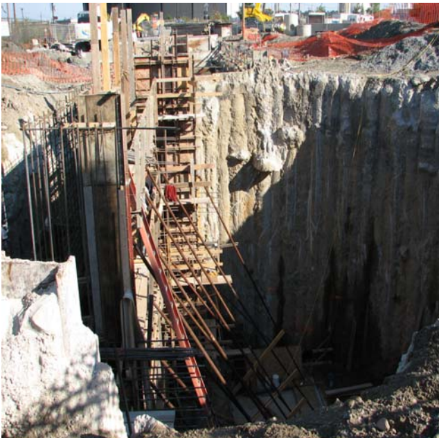
The 067 Gate & Screenings Structure where wet weather flow passes before entering the tunnel through a drop shaft, pumped through the Tunnel Pump Station to the Field's Point Wastewater Treatment Facility.
