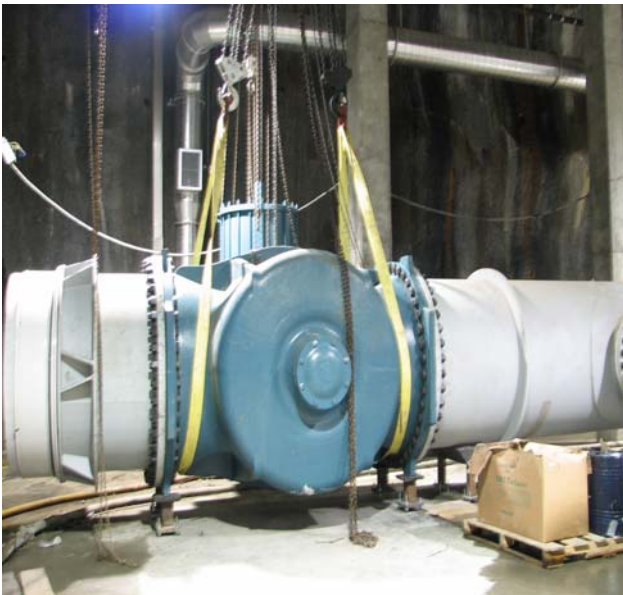
One of the pneumatically controlled valves. The 54" valves control the flow from the Tunnel to Pump Station.
