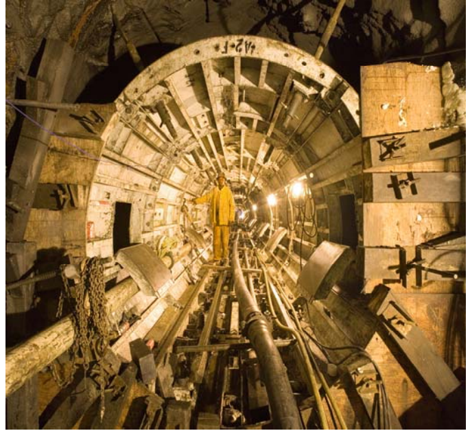
Above, the number 3 Adit concrete forms.
