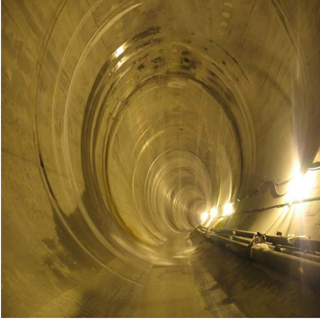
Above, a partial view of the 16,000 foot lined tunnel. The tunnel is 26 feet in diameter, in bedrock.
