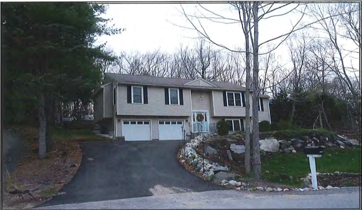
393 CAMP DIXIE ROAD - COMPRESSOR STATION MATCHED PAIR 1B
