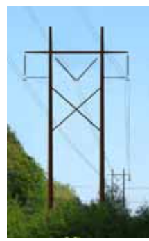
Steel “H” Frame
