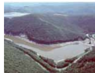
Bear Swamp Pumped Hydro Rowe, MA
