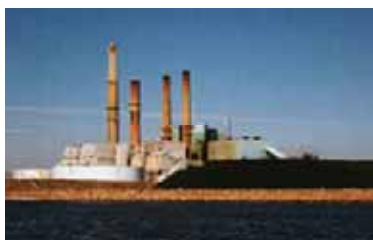
Brayton Pt. Coal/Oil Plant Somerset, MA
