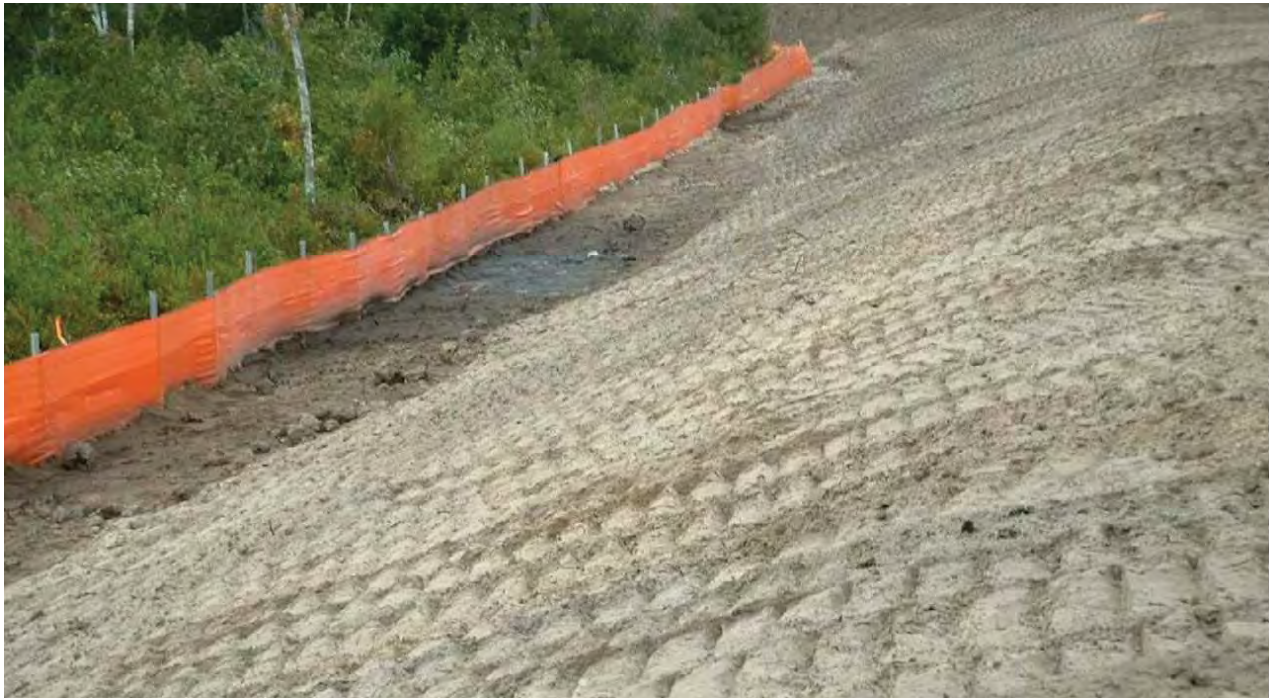
BMP # 37 BARRIER FENCE (CONSTRUCTION FENCE)
