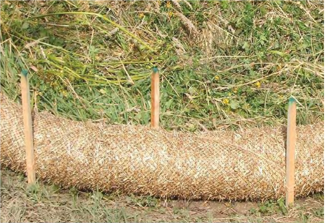
STRAW WATTLE – SHALLOW SLOPE ( \leq 4:1 ) (ALTERNATE STAKING)
