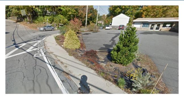
With just this minor widening, tractor trailers (WB-50 design vehicles) appear to have enough room to negotiate this corner without any significant encroachment into the oncoming lane (reference Autoturn diagram 4).
